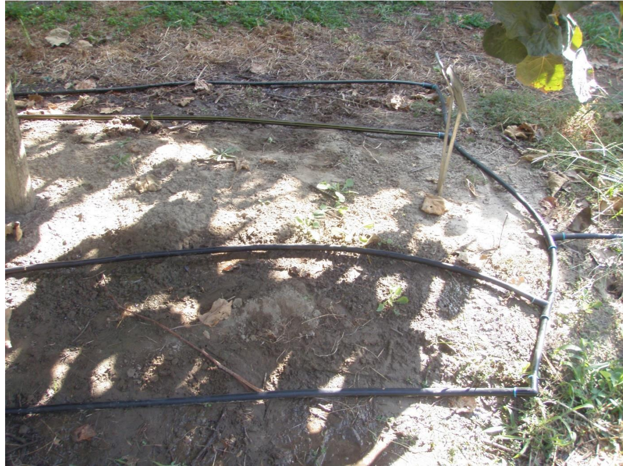
Four line drip system in TRT 02 test plot
